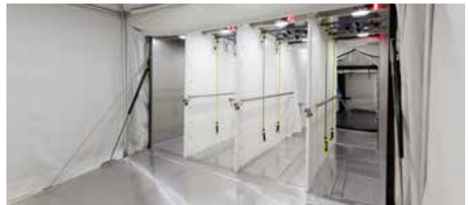
Decon shower lines for ambulatory and non-ambulatory persons - DSAP
